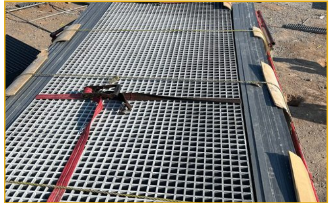
Prepared panels and secure strapping
